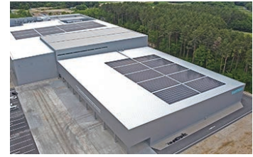
Solar panels at Suntory Kita Alps Shinano-no-Mori Water Plant
