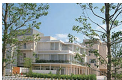
Domyoji-Takadonoen, a general-purpose welfare facility
