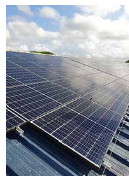
New solar panels installed on the roofs of fermentation facilities
