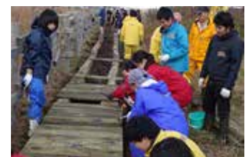
Landscape repair of boardwalk (2014)
