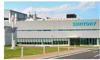
Suntory Products Ltd. Kanagawa Ayase Plant uses rainwater to water plants
