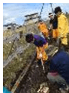
A view of landscape repair
