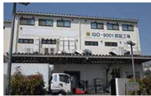
A panoramic view of the Takatsu Plant
