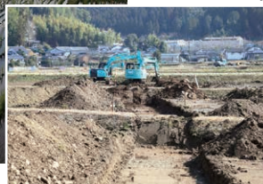
Construction toward recovery
