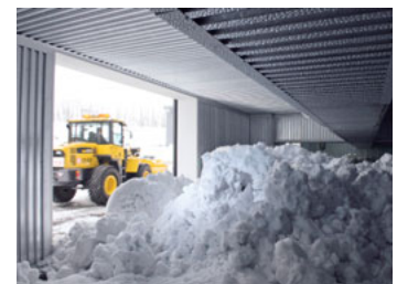
Snow room at the Okudaisen Bunanomori Natural Mineral Water Plant Suntory Products Ltd.
