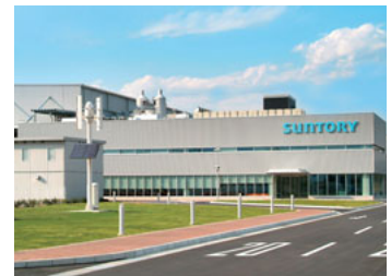
Suntory Products Ltd. Kanagawa Ayase Plant uses rainwater to water plants
