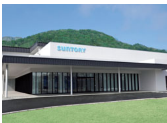
State-of-the-art environmentally-conscious plant Suntory Products Ltd. Minami Alps Hakushu Water Plant
